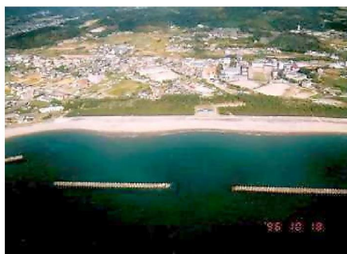
Segmented detached breakwater scheme
